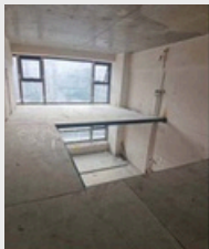
MGO – Structural Base Floor
